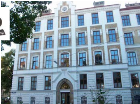
New Middle School, Schopenhauerstraße 70, Vienna 18,
